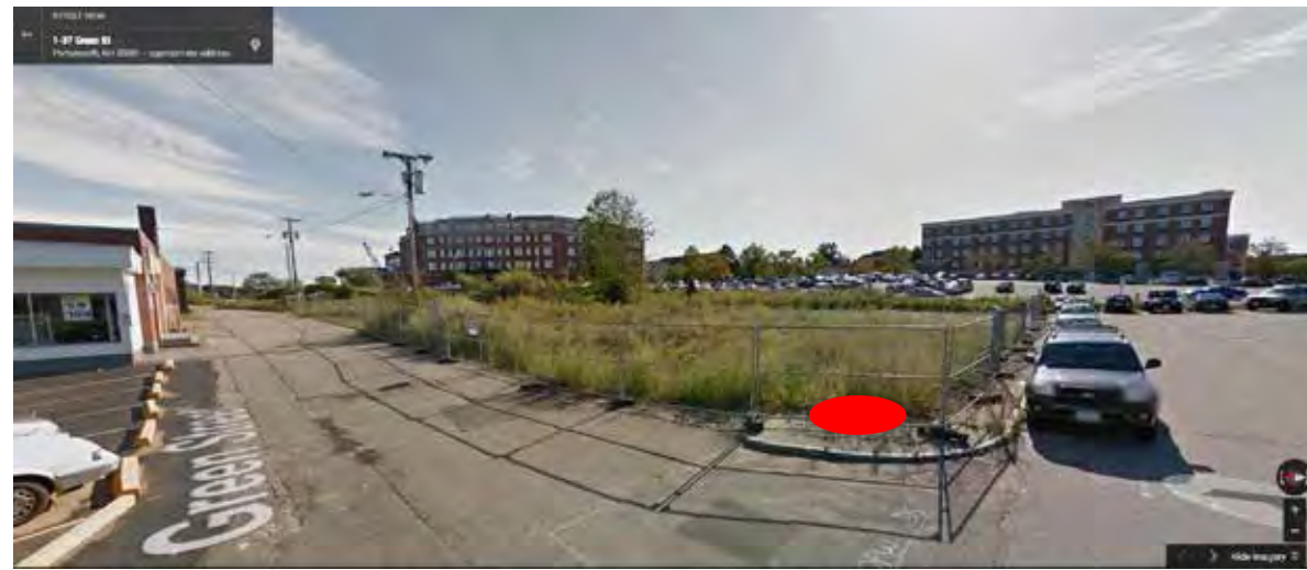
514 Under Construction. Locate in Field with City of Portsmouth
